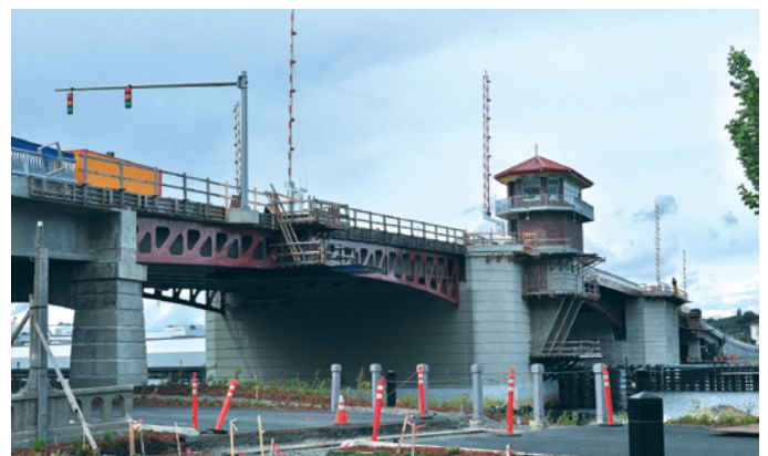
Bridge Construction in 2014 - Photo by Joe Mabel, CC BY-SA 3.0, https://commons.wikimedia.org/w/index.php?curid=32825583
